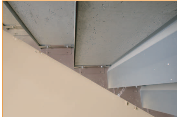
left: Step treads can be tinted to blend into a uniformed look, matching the gray finish above: Back side attachment
